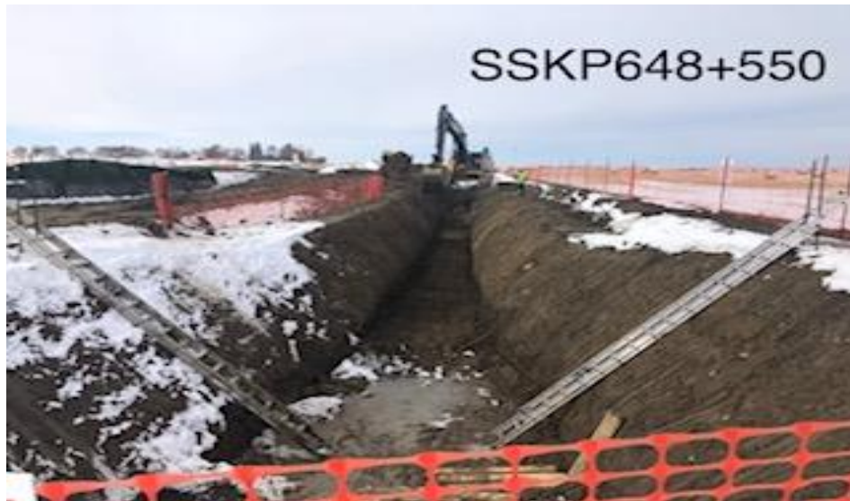
Bell Hole excavation
