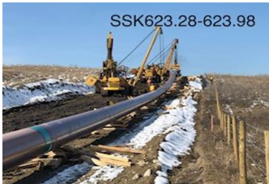
Side booms used to put Section onto rollers in preparation for pull
